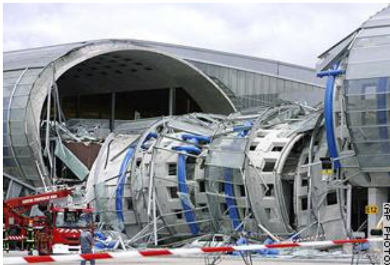
Fig.12 Terminal Roissy Airport Paris – Shell collapse (2004)
