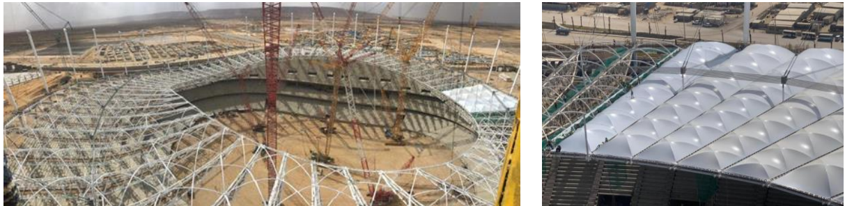
Figure 19: Membrane and arches installation
